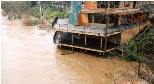
2005 flood—Riverside Inn, Grants Pass, OR
