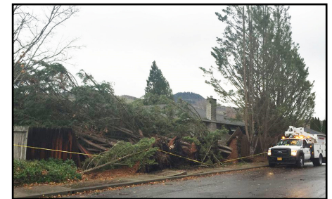
Bryson Way, Medford during December 2014 windstorm Photo courtesy of KDRV NewsWatch 12
